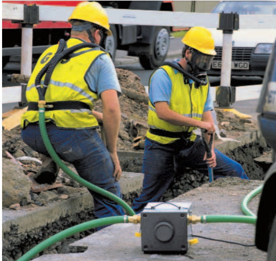
Turbo-Flo assisted fresh air hose breathing apparatus
