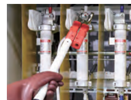
When you push the rope, clip is closed.
