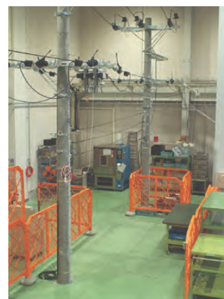
Simulated power pole for electricity distribution line
